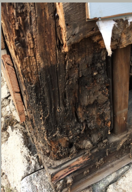
In the Loring Parsonage the ends of corner posts were rotted away or very weak.
