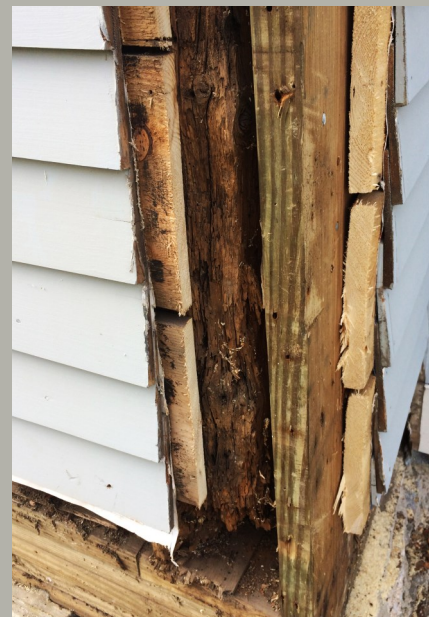
In the Loring Parsonage the ends of corner posts were rotted away or very weak.
